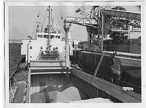
Figure 8: Stone Boat Loading by Conveyor - 1975
