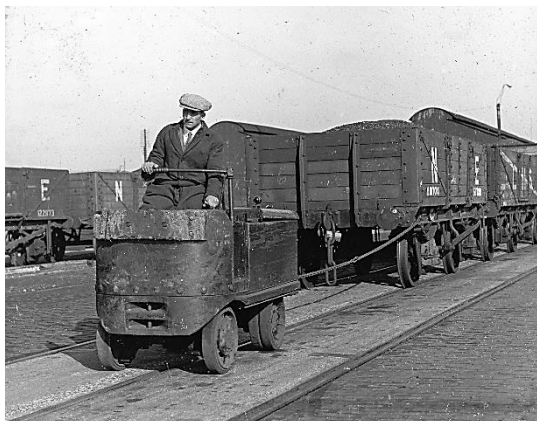
Figure 7: Battery-Electric Trolley Source: Southampton CC Record Office
