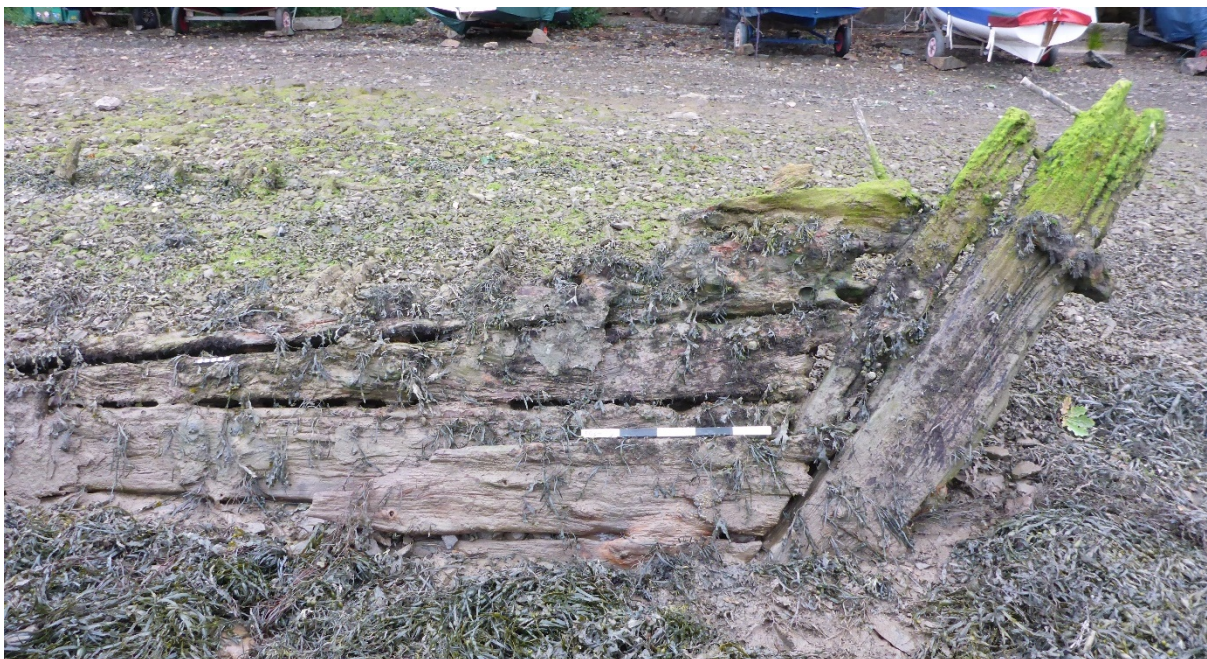
Figure 37: Stern of the Glory including stern post and gudgeons and external planking
