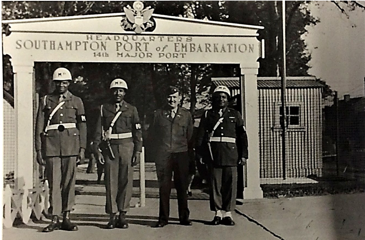
Figure 14: Temporary Gate, Southampton
