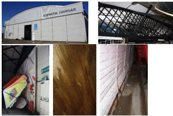
FIGURE 22: TOP LEFT: SOPWITH HANGAR. TOP RIGHT: SURVIVING TIMBER ELEMENTS. BOTTOM LEFT: SLIDING DOORS. CENTRE: WOODEN FLOOR.
