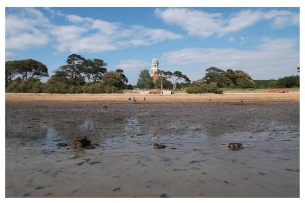
Figure 8. View from the water's edge north-east towards the pier entrance along the central axis of the pier. A complete bent of pilings is visible in the foreground with a spacing of eight foot between piles.
